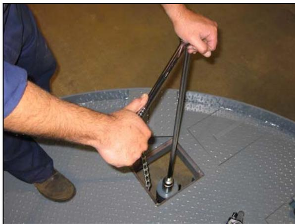
Figure 4 Example of a leveling leg being manually adjusted from the top of the lifting platform via a special access cover.
